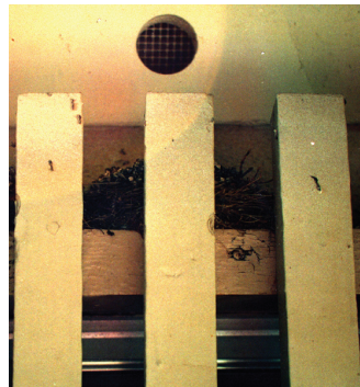
A typical bird's nest on a louver in the base housing area.
